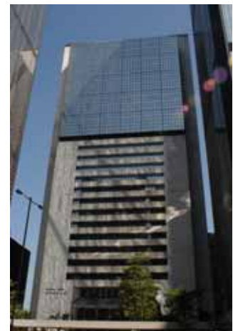
Wanchai Tower of HK Government Building – 3 BIPV Systems
