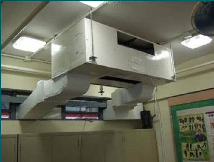
Heat Recovery Ventilator (reclaim ~40% energy)
