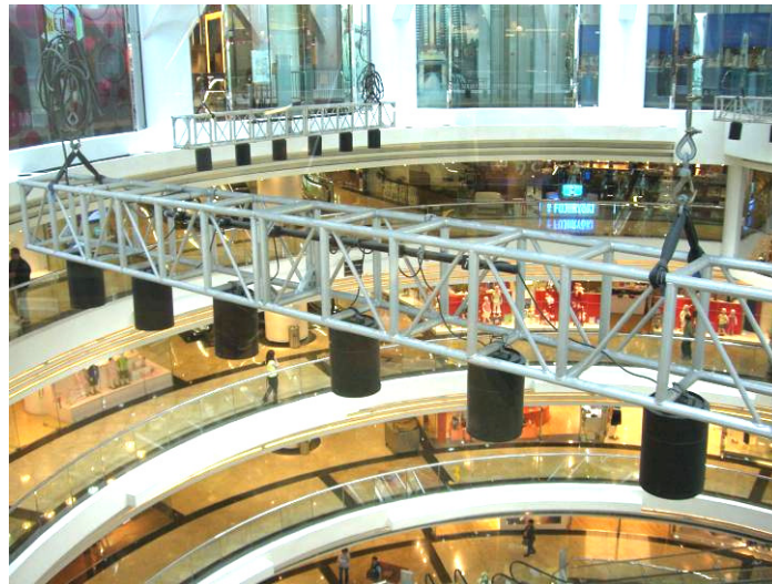
Figure 1.18 Triangulated Frame
