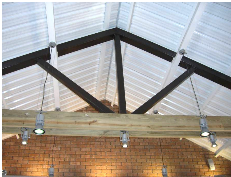
Figure 1.12 Plane Frame – Roof Truss
