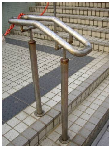
Figure 1.45 Hand rail made of stainless steel
