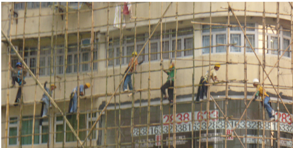
Bamboo scaffolding used in buildings
